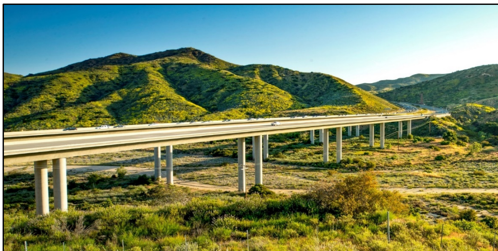
Figure 2 - Elevated segment of SR-241. (Used with permission of the Transportation Corridor Agencies.)
