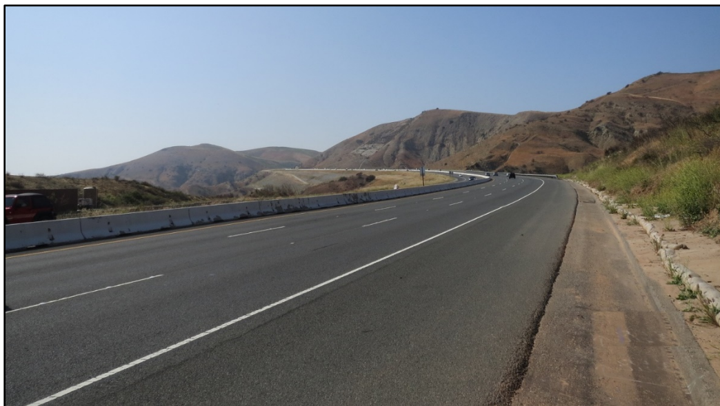
Figure 4 - SR-241 northbound, north of SR-261 interchange. (Photo by 2020-21 Orange County Grand Jury)
