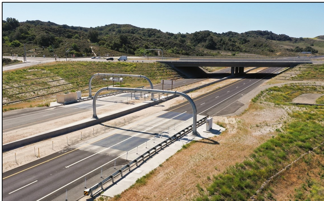
Figure 12 - SR-241 southbound termination at new Oso Parkway Bridge. Los Patrones Parkway surface road begins after the bridge. (Used with permission of the Transportation Corridor Agencies.)
