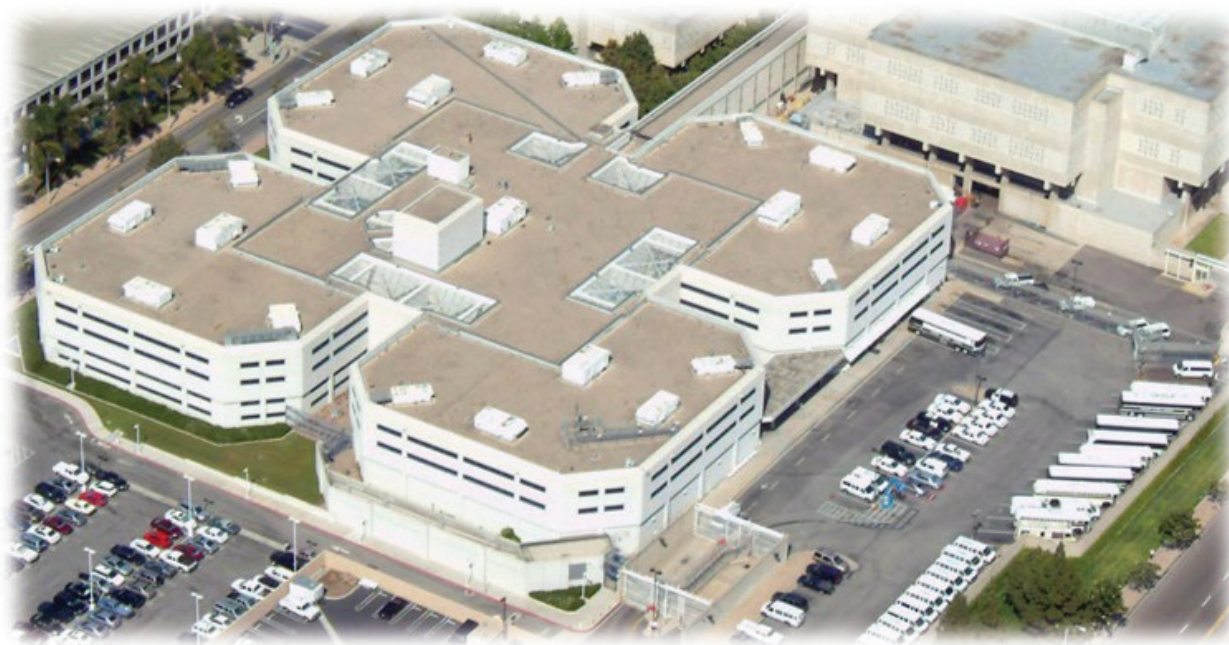
Figure 1 - Overhead view of OCSD Intake & Release Center
