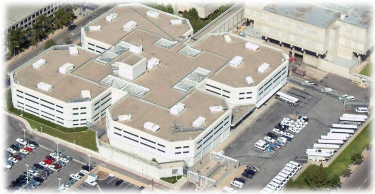
Figure 1 - Overhead view of OCSD Intake & Release Center
