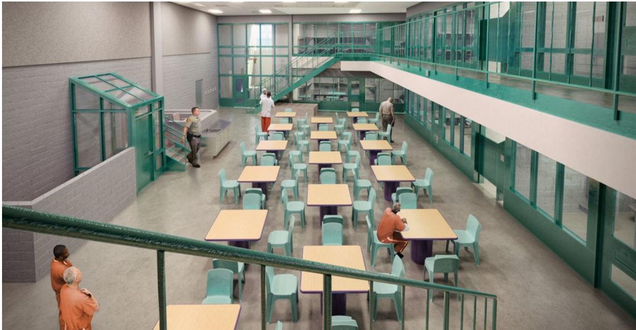
Figure 4 - Typical inmate module at James A. Musick Facility
