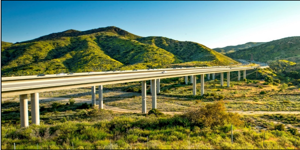
Figure 2 - Elevated segment of SR-241. (Used with permission of the Transportation Corridor Agencies.)
