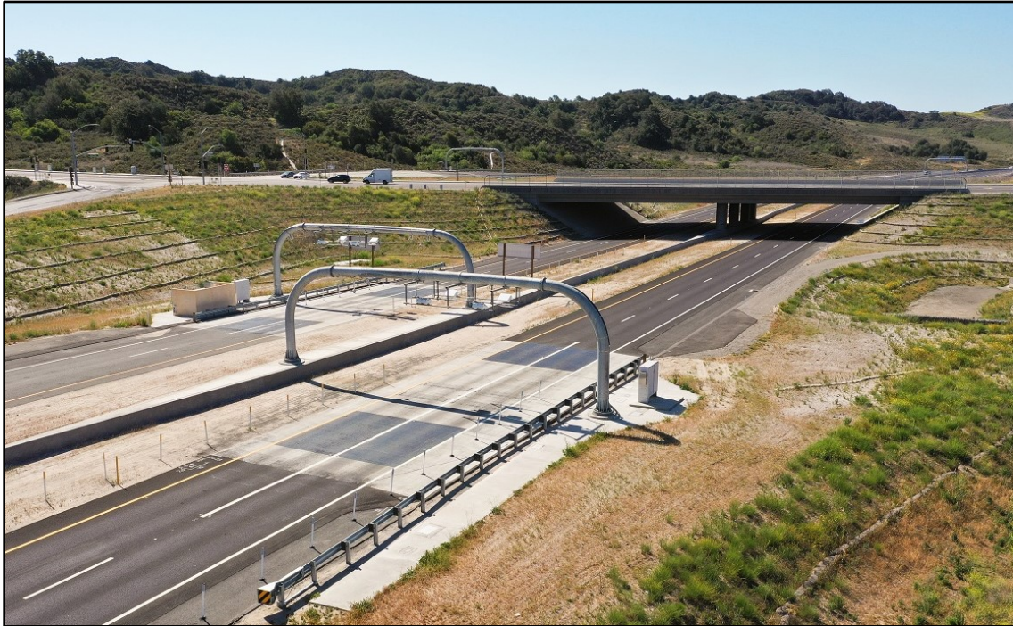
Figure 12 - SR-241 southbound termination at new Oso Parkway Bridge. Los Patrones Parkway surface road begins after the bridge. (Used with permission of the Transportation Corridor Agencies.)
