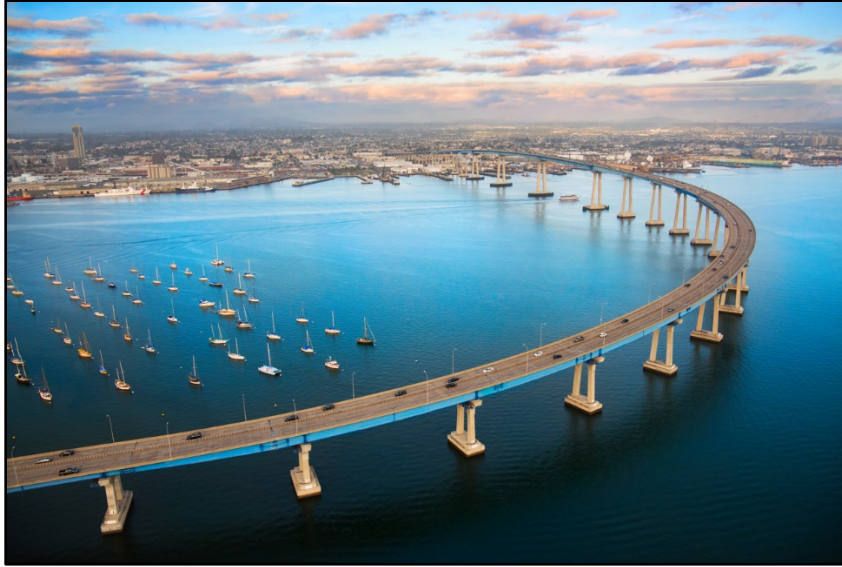
Figure 5 - San Diego - Coronado Bridge. (Not part of The Toll Roads.) Toll collection on the bridge ceased after payoff of construction bonds. (Used with permission ©2021 Art Wagner – Getty Images.)
