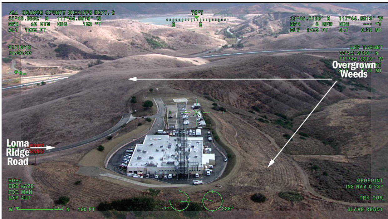
Figure 2: Emergency Operations Center – Aerial View – showing areas where there are dried, overgrown weeds.
