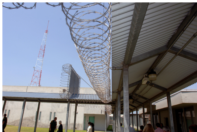
Part of the Theo Lacy Facility in Orange, CA
