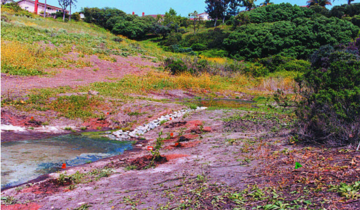
Recently Constructed Wetlands in Laguna Niguel to Filter Urban Runoff into J03P02 Storm Drain that Empties into Aliso Creek ( View 1)
